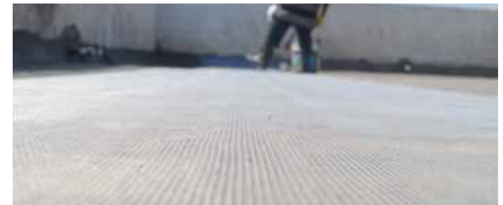
Step 2: Laying of fibre glass fabric
