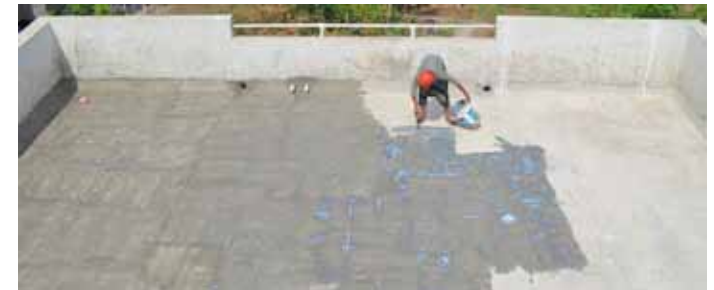
Step 2: Applying the base coat
