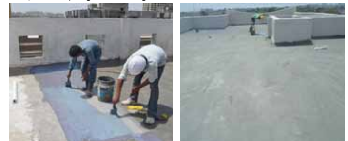
Step 2: Applying 1st and 2nd coat over the fabric
